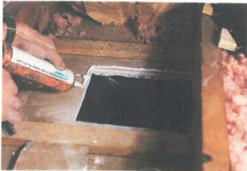
Sealant prevents moisture from leaking into the attic. A thick bead of sealant around the perimeter of the hole creates an airtight bond between the fan's flange and the drywall. Place the fan in the hole carefully, and make sure it sits flat on the ceiling and sealant.
