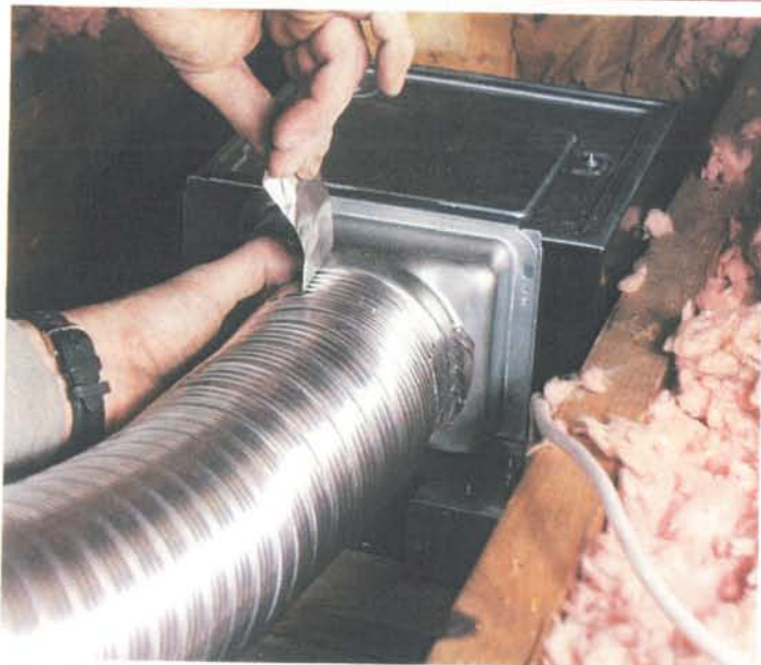
Seal all ductwork tightly. The duct is slipped all the way onto the fan's exhaust port and sealed airtight with aluminum duct tape. Don't use common fabric-backed duct tape, which will deteriorate with time.
