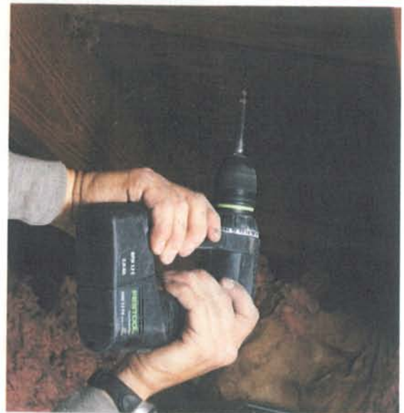
A screw marks the spot on the roof. A screw driven into the center of the traced circle and through the roof sheathing marks the center of the duct and transfers the vent location to the roof where the hole will be cut.
