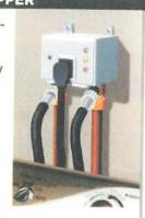
close the valves when a machine is not being used. But most people don't bother. Fortunately, there are devices that will do it for you. The Intelliflow (about \$150), above, senses when the washer is turned on and automatically opens the water-supply valves. At the end of the cycle, it shuts them down. A floor-mounted sensor also closes the valves if it detects water pooling at the washer's base.
