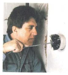
Working from inside, spin the vent brush a few inches into the duct leading outside, then pull it back and clean off the bristles. Repeat until the bristles reach as far as the exhaust hood on the outside wall. (Don't try to shove the lint out with the brush; you may create a clog.) Then go outside and make sure the vent hood isn't plugged. If need be, remove the hood, clean it out, and then put it back.
