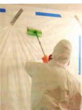
Clean vertical surfaces, too. Interior walls should be covered in plastic. This way, the surface can be wiped, vacuumed, and thrown out at the cleanup stage, eliminating the chance of lead dust remaining on the wall.
