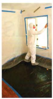
Shrink the containment zone. The 10-ft. containment zone used outdoors shrinks down to a single zone of only 6 ft. for indoor work. Fitting your tools and waste in this small area can be tough. If you can, find a helper so that you can hand off contained waste.
