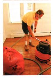
Make a final pass. After vacuuming off your coveralls and disposing of the plastic, do one more pass with the vacuum. Finish up with a wetcleaning cloth, which should be used to wipe no more than 40 sq. ft. before being replaced with a fresh one.
