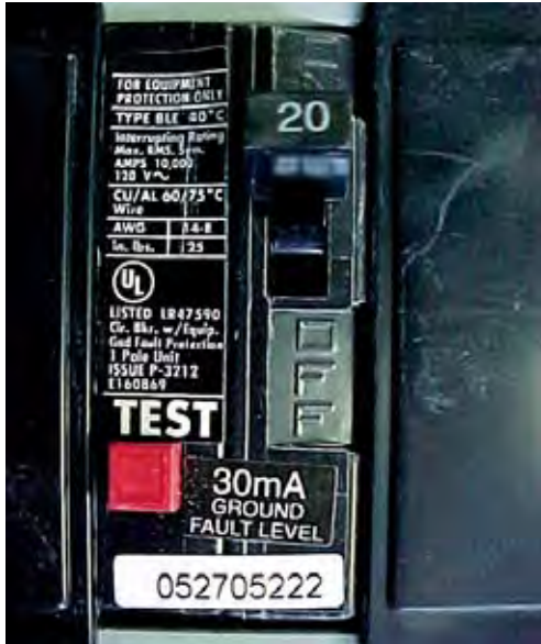
GFPE Circuit Breaker
