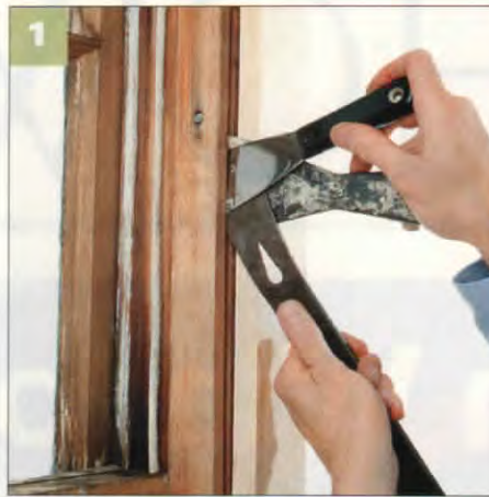
To pry off a stop molding, first score the paint or varnish at any joints. Next, carefully insert a broad putty knife into the joint and put a second knife behind it. Then slide a flat prybar (1) between the knives. While the knives protect the wood, carefully pry off the moulding near any nails. When the stop is loose, carefully bow it (2) to release the ends. Watch for miters and pockets.
