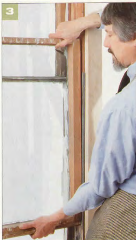
With one stop off, there's enough clearance to lift and angle the sash out of the window (3). Before removing the sash, secure the weight with a knot or clamp (4); the cord end can easily pop out of the sash stile (see arrow, above).
