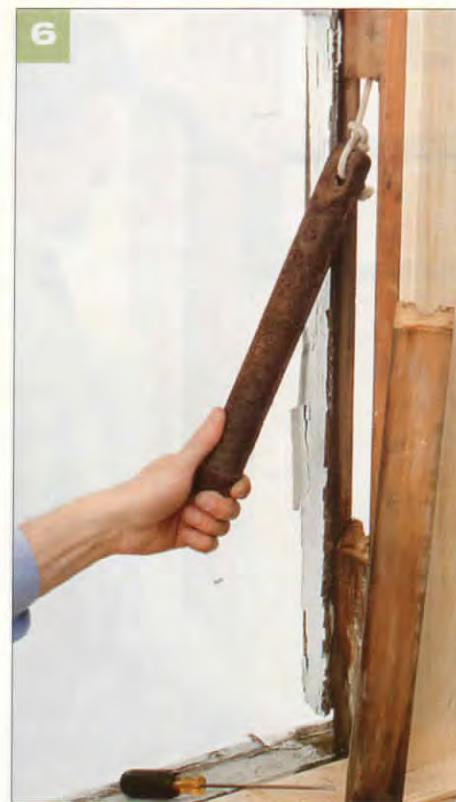
To remove the parting bead, grasp it with locking pliers (5), then work the strip out from the notch in the upper sash meeting rail. Note that the bead may already be weak or worn at this point. Angled ends and a single wood screw secure the weight pocket door (6) and access to the weights.
