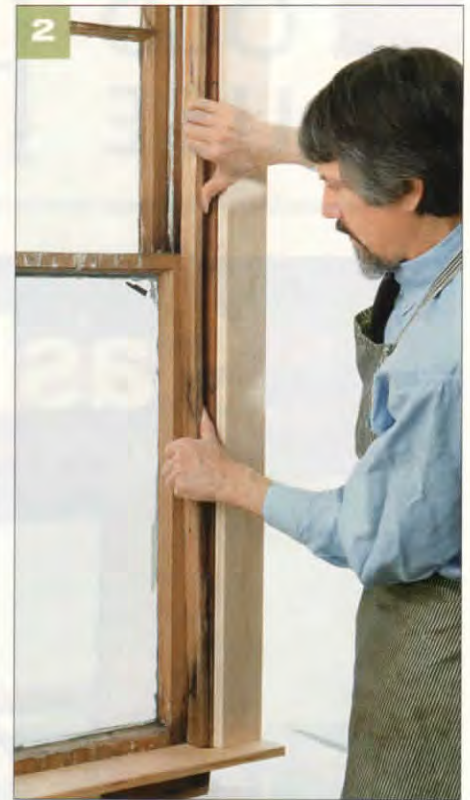
To pry off a stop molding, first score the paint or varnish at any joints. Next, carefully insert a broad putty knife into the joint and put a second knife behind it. Then slide a flat prybar (1) between the knives. While the knives protect the wood, carefully pry off the moulding near any nails. When the stop is loose, carefully bow it (2) to release the ends. Watch for miters and pockets.
