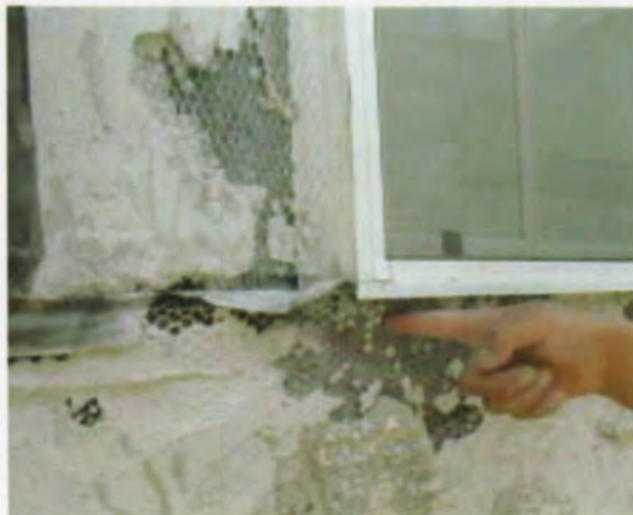
Figure 3. Undersized or omitted diverter — or kickout — flashings allow water to flow beneath the cast-stone facade (above). Window flanges that lap under instead of over building paper can bring rain water into direct contact with the sheathing (right).
