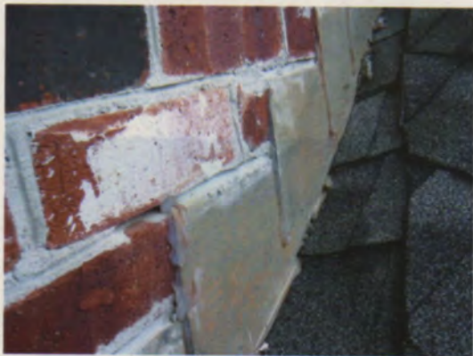
Figure 2. Stepped counterflashings installed in mortar joints (above) are no better than saw-cut flashings at diverting water from the cavity — unless they happen to run through to the sheathing and tuck under the building paper, which is rare. The work often gets sloppier where the installer thinks no one will see it, as in this bungled mishmash of surface-applied metal (right).
