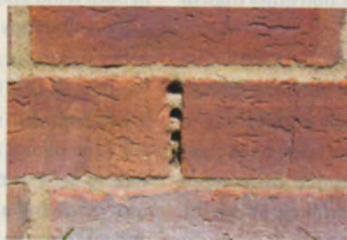
Figure 7. Randomly placed weeps (top) serve no purpose because there's no through-wall flashing to divert the water. Weeps drilled out after the brick is in place are a sure sign of missing flashing (above).
