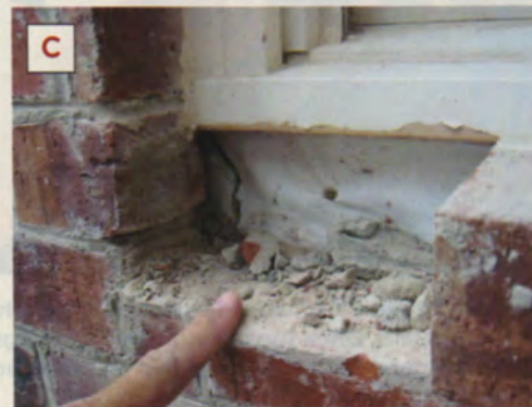
Figure 5. Unlike this one (A), window sills should be sloped 15 degrees. A close inspection reveals potential leak spots along this window frame (B); because there's no through-wall flashing, water will get into the framing. Instead of flashing below this window (C), there's a cavity clogged with mortar and compromised torn housewrap.
