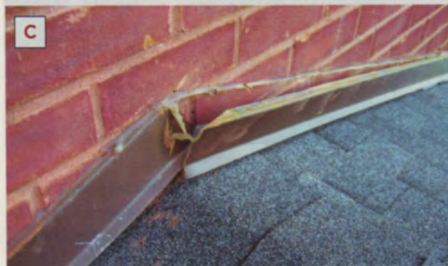
Figure 1. Counterflashings installed in saw-cut kerfs, whether at shed roofs (A) or sloped roofs (B, C), do nothing to divert water from the cavity behind the brick. These installations have a high rate of failure; copious amounts of caulk and the presence of nails or screws are dead giveaways that the flashing is useless. The sketch above, made by the author during a site visit, explains to the client the difference between a kerfed-in and a through-wall flashing.
