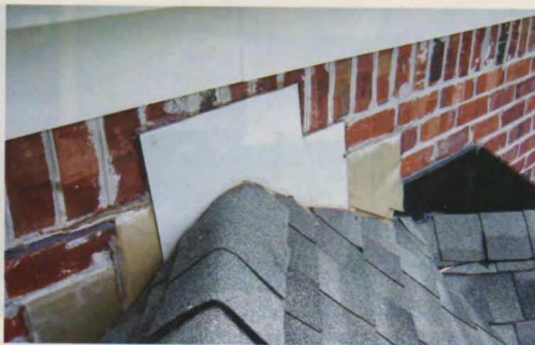
Figure 2. Stepped counterflashings installed in mortar joints (above) are no better than saw-cut flashings at diverting water from the cavity — unless they happen to run through to the sheathing and tuck under the building paper, which is rare. The work often gets sloppier where the installer thinks no one will see it, as in this bungled mishmash of surface-applied metal (right).
