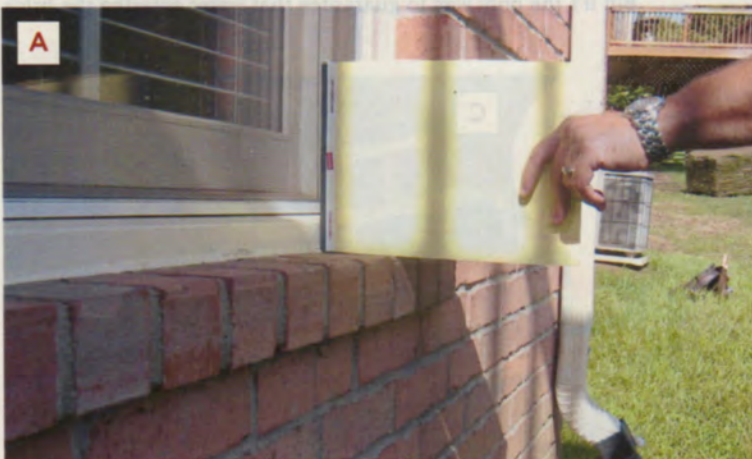
Figure 5. Unlike this one (A), window sills should be sloped 15 degrees. A close inspection reveals potential leak spots along this window frame (B); because there's no through-wall flashing, water will get into the framing. Instead of flashing below this window (C), there's a cavity clogged with mortar and compromised torn housewrap.
