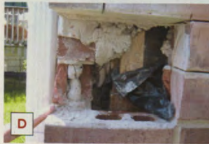
Figure 6. Destructive inspections from inside (A, B) and out (C, D) often reveal the cause of moisture, stains, and mold on interior finishes: The cavity is clogged with mortar, which holds water that eventually soaks the sheathing, framing, insulation, and drywall.
