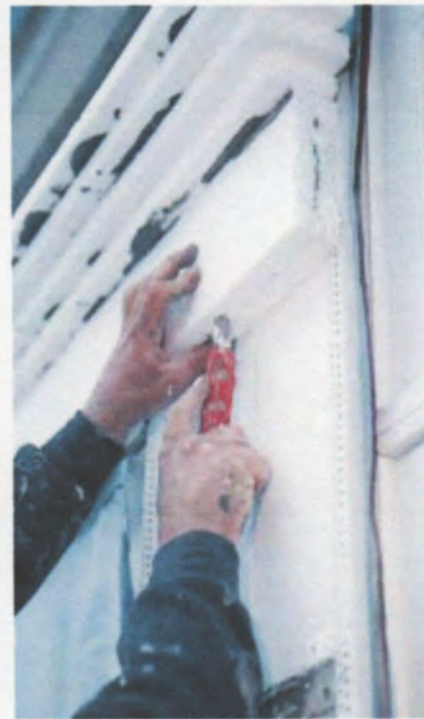
Figure 9. Hand-carved foam details are common in synthetic stucco systems (left). For extra durability, the foam trim is either bedded in mesh tape or capped with vinyl beads, as shown here (right).
