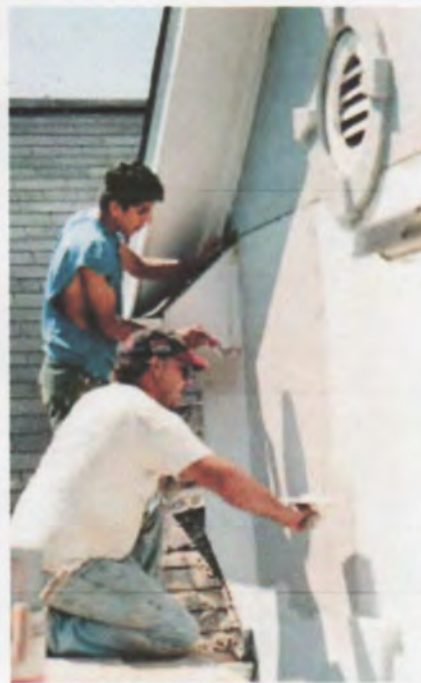
Figure 10. The base coat plaster is first used to bed all joints and to fill inside and outside corners (left). Once the bedding cures, the base coat is troweled onto an entire elevation at one time to avoid cold joints. After the base coat has cured for 24 hours, the finish coat is troweled on and textured, much like conventional stucco (right).
