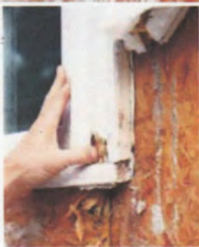
Figure 2. This three-year-old Greensboro, N.C., home was damaged when water leaks around windows and poorly-flashed roof-wall connections became trapped behind the EIFS cladding (above). Even window trim, jambs, and sills were rotted (inset) and had to be replaced.
