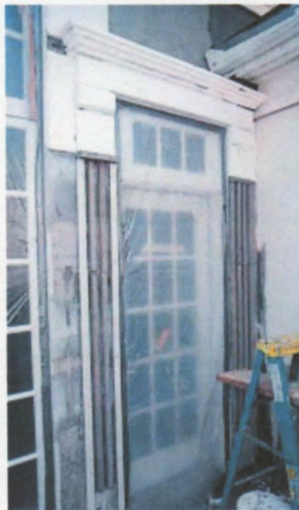
Figure 9. Hand-carved foam details are common in synthetic stucco systems (left). For extra durability, the foam trim is either bedded in mesh tape or capped with vinyl beads, as shown here (right).
