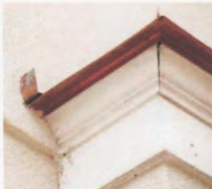
Figure 6. Missing kick-out flashings at roof-wall junctions are a common source of leaks in EIFS failures. The author prefers a heavy-gauge copper for these flashings.
