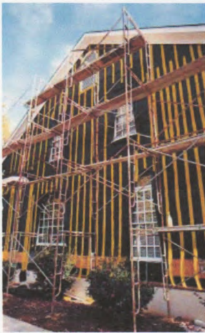
Figure 8. With the drainage plane and scaffolding in place (left), the Durock cement board panels are applied in a staggered pattern (middle). Spaces between panels provide a keyway for the stucco. A vinyl starter bead maintains a clean reveal along the exposed bottom edge of the cement board (right).
