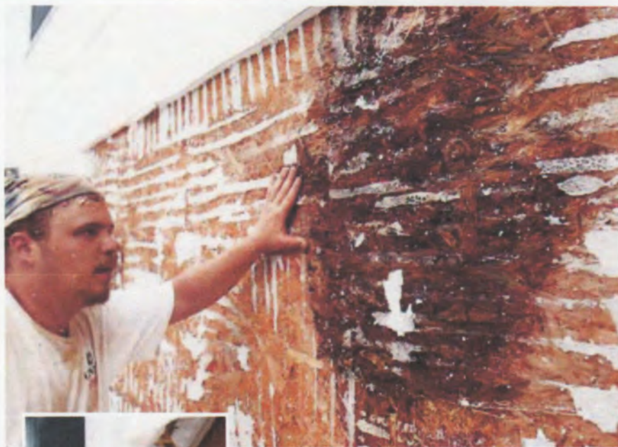
Figure 2. This three-year-old Greensboro, N.C., home was damaged when water leaks around windows and poorly-flashed roof-wall connections became trapped behind the EIFS cladding (above). Even window trim, jambs, and sills were rotted (inset) and had to be replaced.
