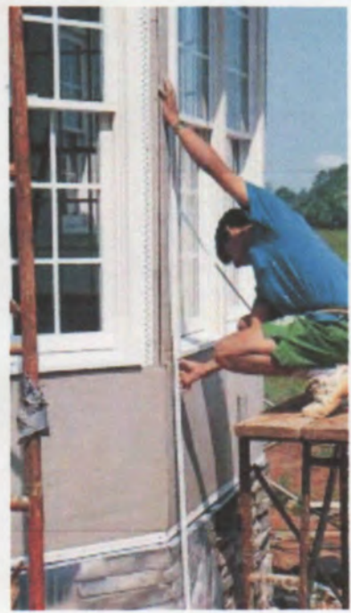
Figure 8. With the drainage plane and scaffolding in place (left), the Durock cement board panels are applied in a staggered pattern (middle). Spaces between panels provide a keyway for the stucco. A vinyl starter bead maintains a clean reveal along the exposed bottom edge of the cement board (right).
