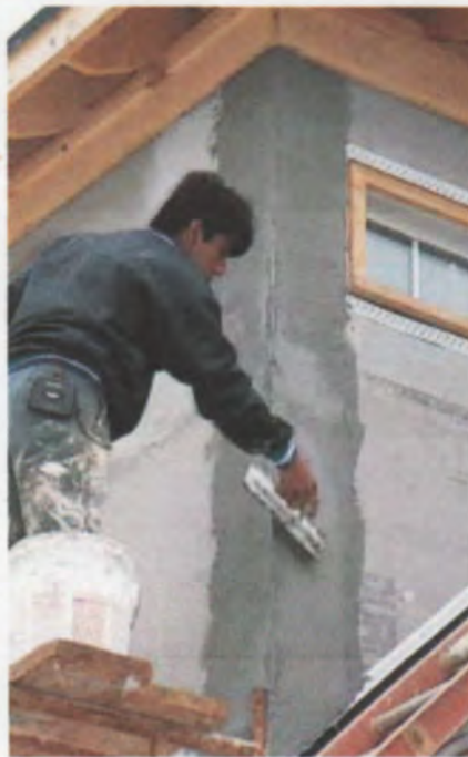
Figure 10. The base coat plaster is first used to bed all joints and to fill inside and outside corners (left). Once the bedding cures, the base coat is troweled onto an entire elevation at one time to avoid cold joints. After the base coat has cured for 24 hours, the finish coat is troweled on and textured, much like conventional stucco (right).
