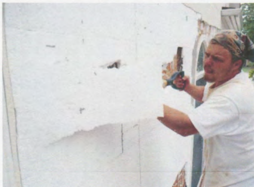
Figure 4. Large sections of foam are pried off with flat-faced shovels; smaller pieces and detailing are removed with spatulas or trowels. A crew is stationed on the ground during tear-off to clean up.
