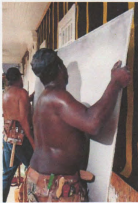
Figure 8. With the drainage plane and scaffolding in place (left), the Durock cement board panels are applied in a staggered pattern (middle). Spaces between panels provide a keyway for the stucco. A vinyl starter bead maintains a clean reveal along the exposed bottom edge of the cement board (right).
