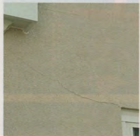
Figure 5. Window corners and narrow intersections between large wall sections are points of stress concentration where cracking may occur. If possible, the design should allow for isolation joints to relieve stress at such locations. In any case, the secondary weather barrier must provide protection for wall materials beneath the EIFS.
