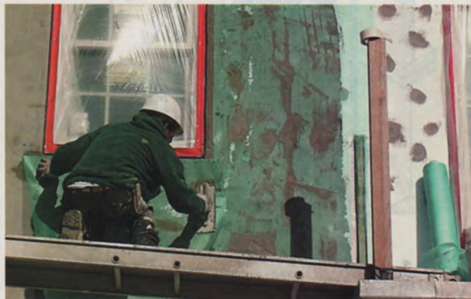
Figure 3. Woven reinforcing mesh (top left) serves to stop the cement and acrylic base coat from cracking. A coating protects the mesh against the alkaline cement, but mesh may still be weakened by moisture and chemical attack. A worker trowels the mesh into the wet base coat (above). For good coverage, the authors recommend applying the base coat in two layers: one layer before troweling in the mesh, and a second layer immediately afterward. Exposed mesh (bottom left) tends to lose strength over time.
