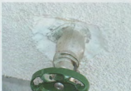
Figure 8. All penetrations should be flashed beneath the EIFS, as well as surface-sealed at the joint. In this example, peel-and-stick membrane is used to seal the electrical box to the housewrap (top left). A gap is left between the EIFS and the box (top middle), and the gap is then filled with backer rod and sealant (top right). Hose bibbs (left) receive a similar treatment.
