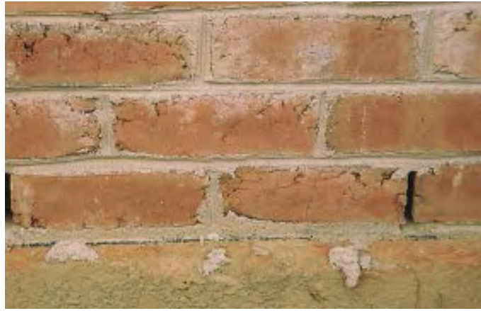
Figure 9. The most dependable type of weephole is the open head joint.
