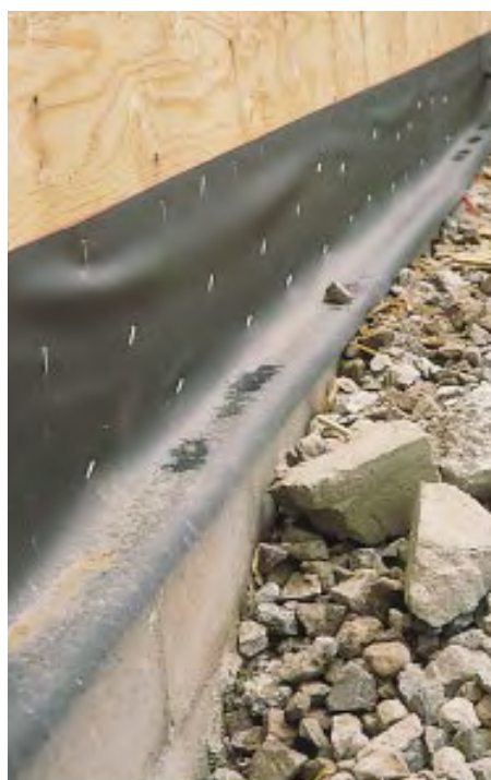
Figure 2. Through-wall flashing and weepholes direct water in the air space to the exterior.
