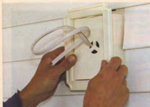
Utility boxes create receiving channels. A snap-on molding holds panel ends around a light box near the front door.
