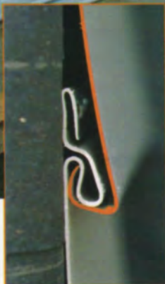
Pushing up locks panels together. The bottom edge, or butt, of one panel clicks into the locking channel at the top of the preceding course, and the siding goes up.
