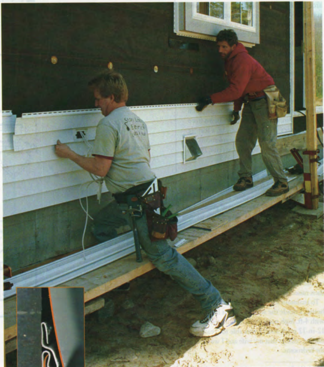
Pushing up locks panels together. The bottom edge, or butt, of one panel clicks into the locking channel at the top of the preceding course, and the siding goes up.
