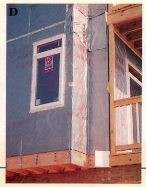
has direct access to the structure. A leak at this point may never show up inside the house, but can nonetheless lead to rot over time. Make sure your housewrap extends all the way around corners. We typically add a layer of tarpaper over the housewrap behind all corner trim boards.
