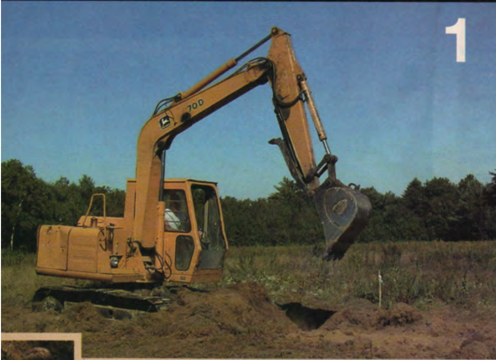
A FEW WEEKS LATER , the excavation contractor got to work. In a matter of minutes, he dug a room-size hole for the new septic tank. INSET: As the first step in any septic system design, the soil at the proposed site must be evaluated. Here, a soil scientist analyzes a test pit. By observing the various layers and matching the dirt to a color-coded key, he is able to determine the type of soil, how well it drains, and the location of the seasonal high-water mark, which establishes the limit of a leach field's depth.
