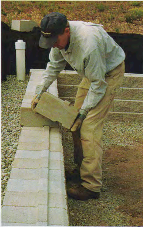
Weatherproof shims handle minor adjustments. For long stretches of wall, the author finds the work goes quickly (photo left). But slowdowns are inevitable. When the tops of adjacent blocks deviate by more than \frac{1}{32} in., adjustments may be required. When blocks have to be shimmed, the author uses narrow pieces of sheet aluminum that won't corrode, rot or wash away over time (photo above).
