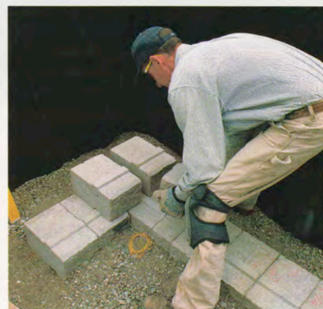
Inside corners are woven. The author sets an inside corner on the first course of block, establishing the spacing for a woven pattern to give the corner interlocking stability.
