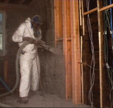
must first air-seal any penetrations (can lights; holes around pipes, ducts, and cables; and the gap around chimneys) before blowing. Loose-fill settles about 10% after installation, so this must be accounted for when planning how deep to blow in the insulation.
