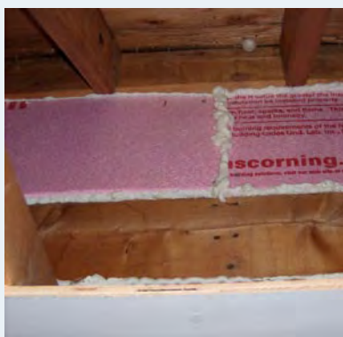
Figure 7.1. When researchers pulled back the porch ceiling, they found the wall board was missing so nothing was covering the insulation on this exterior wall. An air barrier of rigid foam board was put in place with spray foam (Source: Moriarta 2008).
