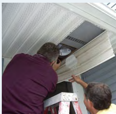
Figure 7.1. When researchers pulled back the porch ceiling, they found the wall board was missing so nothing was covering the insulation on this exterior wall. An air barrier of rigid foam board was put in place with spray foam (Source: Moriarta 2008).
