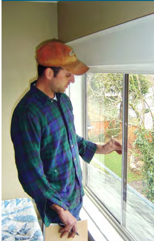
(left) Auditors will check for dry rot and moisture problems as well as air leakage.
