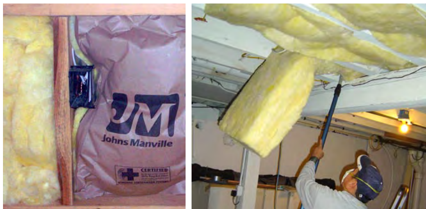
Figure 1.1. (left) Cut fiberglass batt insulation to fit around electrical boxes and wiring or pipes that run through the walls. Compressions like these ruin the batt's thermal alignment with walls and lessen its effectiveness.
