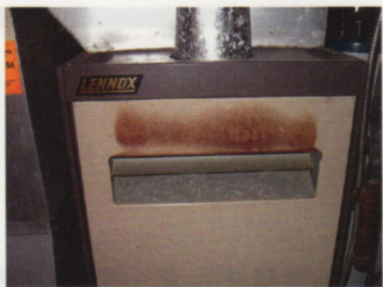
The staining is evidence of backdrafting as a result of negative air pressure in the home.
