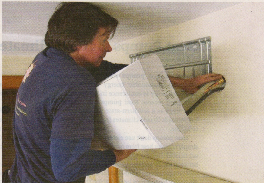
Chris Blaisdell of ReVision Energy mounts an indoor unit in a finished basement. Compared with the blower needed to move air through a ducted system, the small fan in this unit uses very little electricity.
