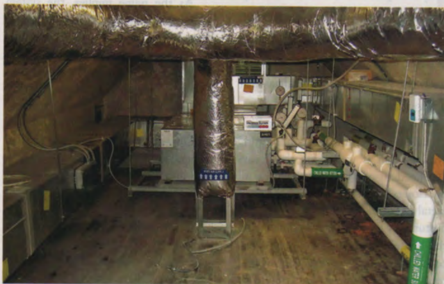
The system's air handler and trunk lines are easily installed in extra attic space.
