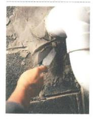
Hydraulic cement is ideal for patching small holes and cracks, even when water is actually flowing through. The material, a powder mixed with water to a putty-like consistency, expands slightly and sets within five minutes. The product contains portland cement, a caustic, so wear rubber gloves when applying.
