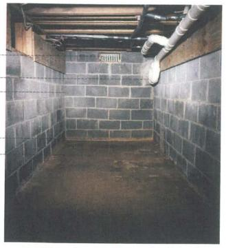
In this basement, the darkened concrete blocks offer a clue that water is seeping through the foundation walls. If incoming water can't be diverted from the outside, the owner will need to find ways to block its entry from the inside.
