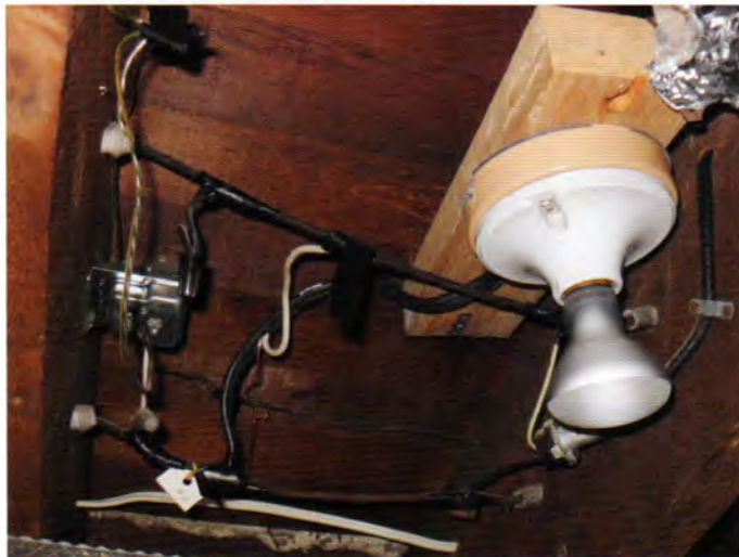
Here is an incorrect connection with newer wiring and the shiny black tape. This should be in a junction box.
