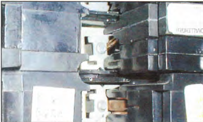
Fig. 8 - E Stab in F Socket
