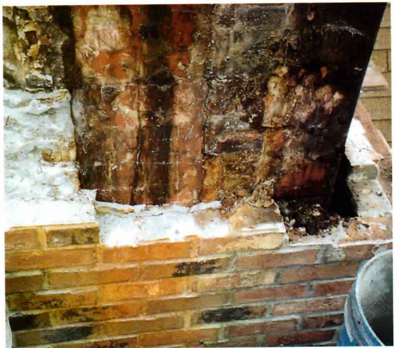
Figure 6. On removing a loose brick during a repair, the author discovered that the standard mortar used to set the flue liners had eroded (above), allowing creosote to leak in between the liners and the chimney wall (right). Flue liners should be set in non-water-soluble refractory cement.
