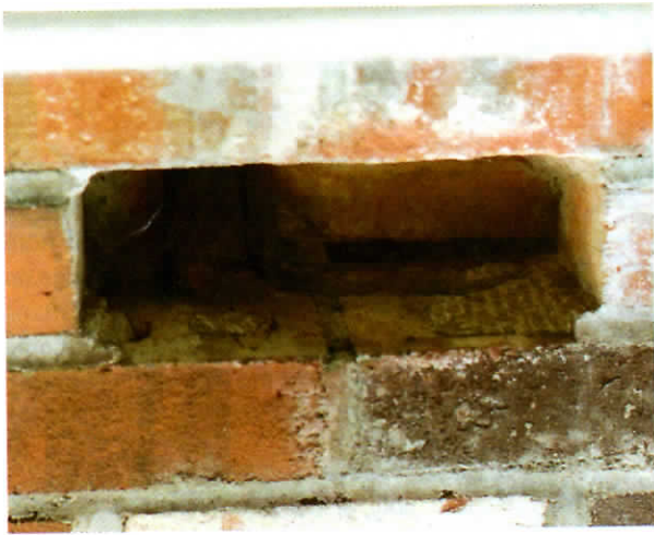
Figure 6. On removing a loose brick during a repair, the author discovered that the standard mortar used to set the flue liners had eroded (above), allowing creosote to leak in between the liners and the chimney wall (right). Flue liners should be set in non-water-soluble refractory cement.
