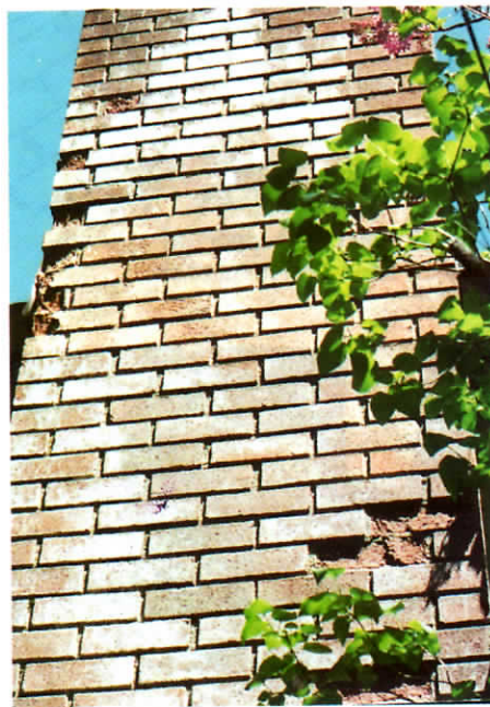
Figure 7. The decorative, deeply raked joints in this chimney allowed water to pool and soak into the brick. When the saturated brick was exposed to extended sub-freezing temperatures, the water froze and expanded, causing the brick to spall.
