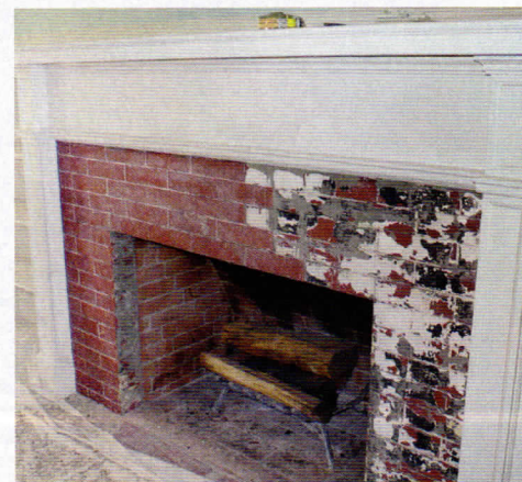
ABOVE Never paint a brick or stone surround—or a future owner may be forced to do this. LEFT Blue Bear's Soy-Gel removes paint from masonry safely and easily.
