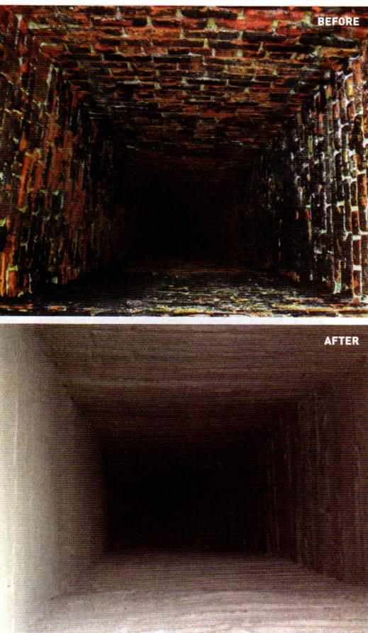
TOP Clay flue liners made by Superior Clay. LEFT An old square flue before lining; the same flue, after being lined using the Thermocrete process.
